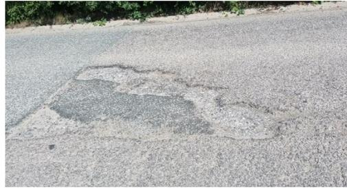
The pothole at the site exit onto the A120 needs repair again and the directional bollard has been damaged and needs replacing/repairing.
